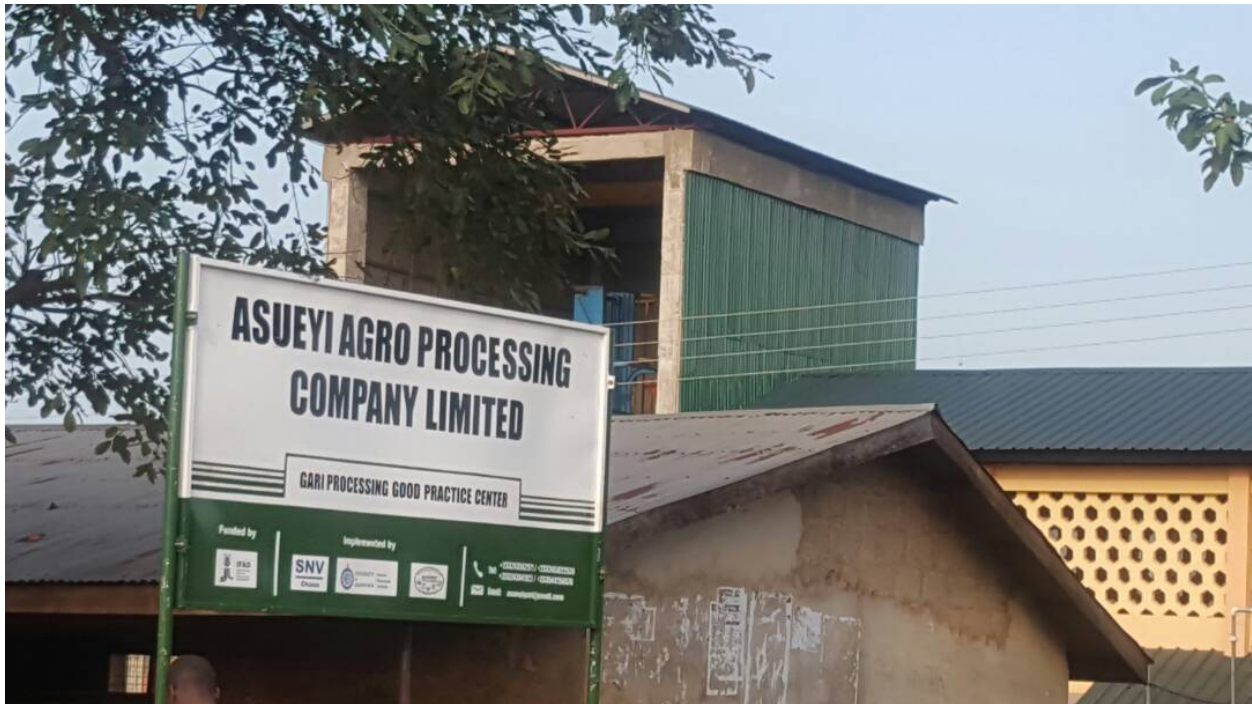
PREMISES OF THE GASIFICATION PLANT (ASUEYI)
