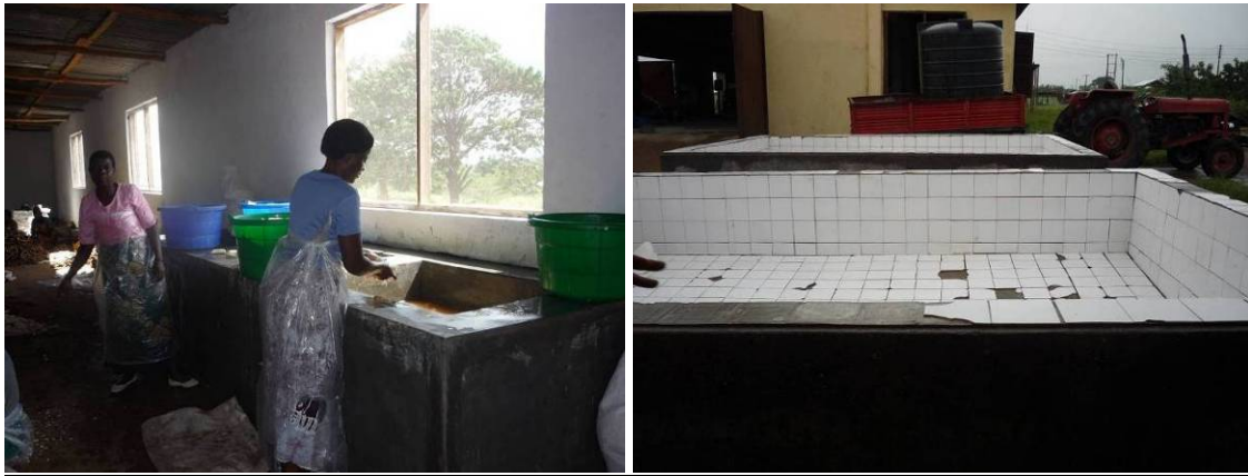
Figure 12: Acceptable (left) washing/soaking facilities vs unacceptable (right) washing facilities
