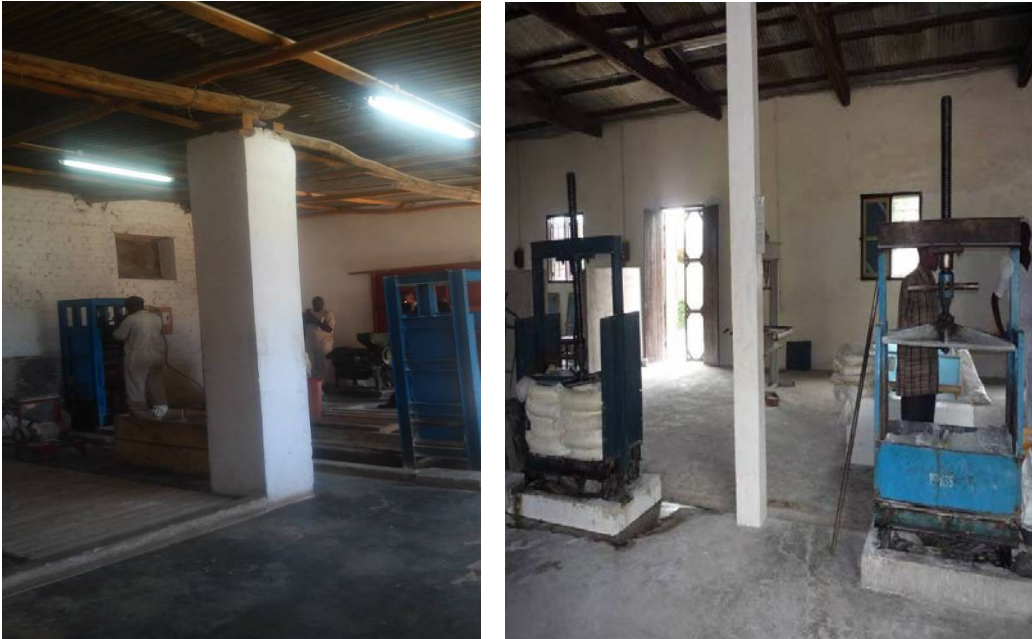
Figure 36: Two upgraded processing plants (left and right) showing wet processing layout with dewatering for HQCF and gari respectively
